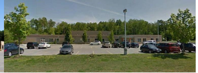
St. Noel Catholic Elementary School
